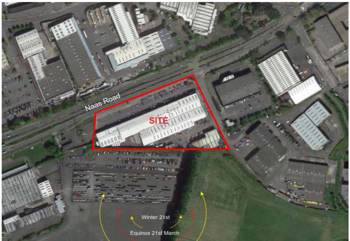
Figure 1: Aerial View of the subject site
